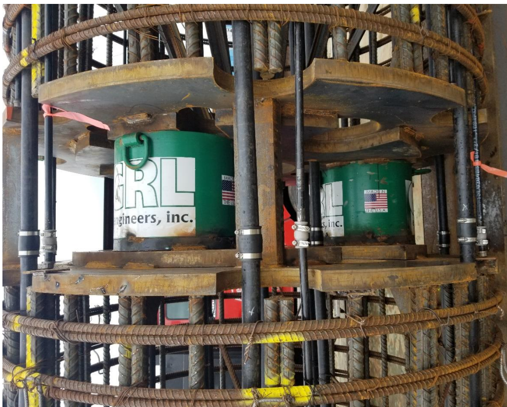
Figure 4. 20 MN Bi-Directional Jack Assembly Attached to the Reinforcing Cage.
