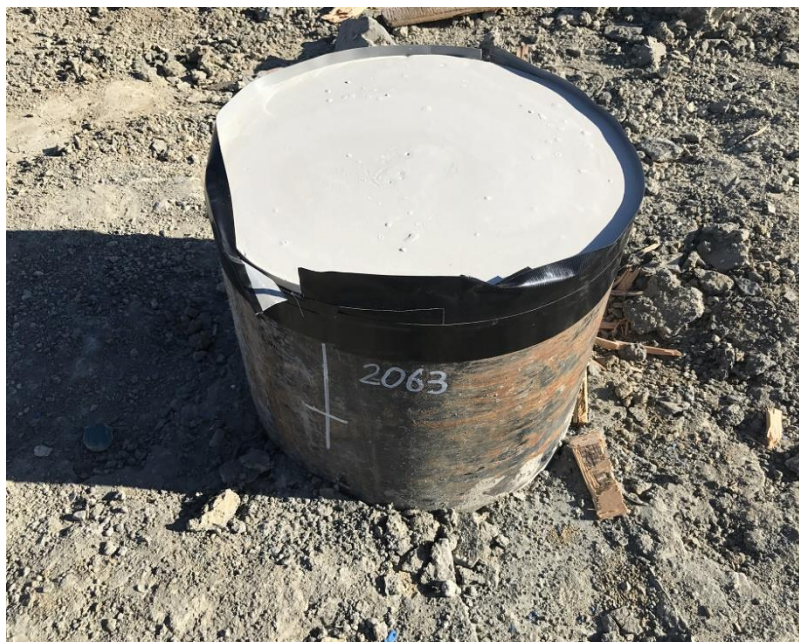
Figure 2 Pile top leveling
