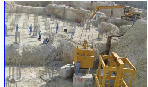
Foundations for Convention Tower, Qatar
