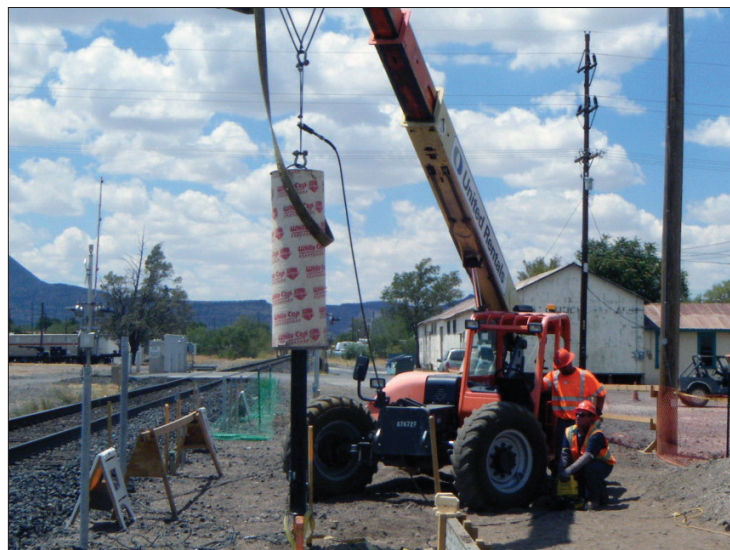
Figure 1. Drop hammer with pile extension (photo courtesy Atwell, LLC)
