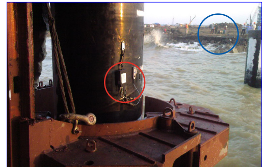
Red circle: Wireless sensors attached to pile; Blue circle: Engineers conducting the test with the PDA model PAX
