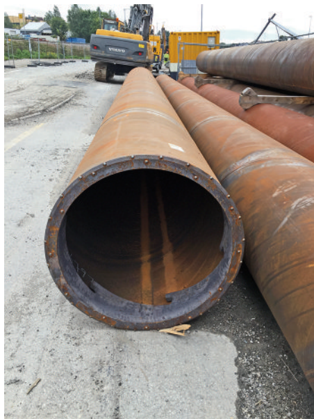
(L) Button driving ring at tip of pipe pile and (R) bottom of a DTH to fit inside pipe pile
