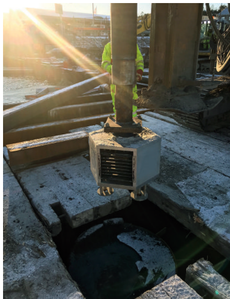
Attachment of the device to the end of a drill string
