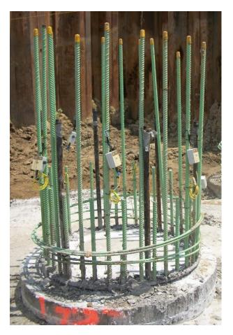
Figure 1. Thermal wire cables attached to data loggers
