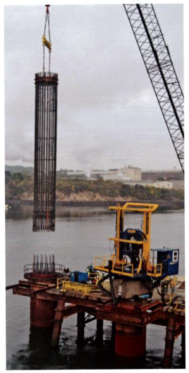
Figure 11: Reinforcing Steel Cage Placement.
