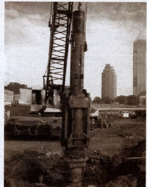
GRL's 3 tonnes Hammer with Cleveland Skyline
