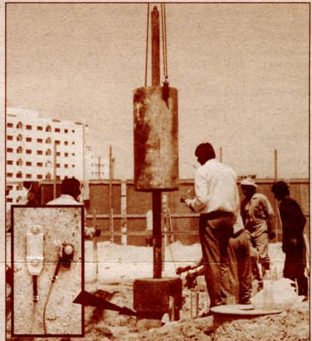
PDA test of Drilled Shaft (Photo courtesy of Dr. M. Mukaddam, I&M, Dubai, UAE)
