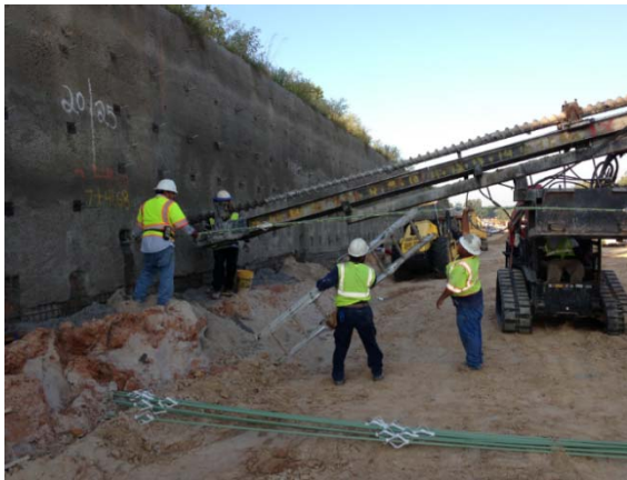
Figure 2: Excavator Mounted Drill Attachment
