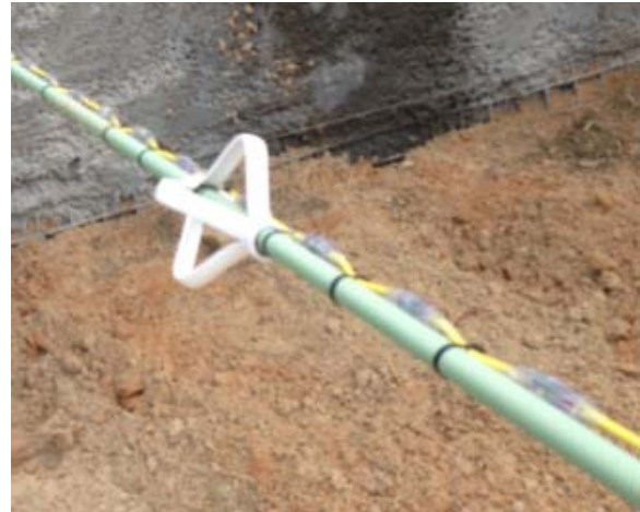
Figure 7: Thermal Wire Affixed to Tension Bar
