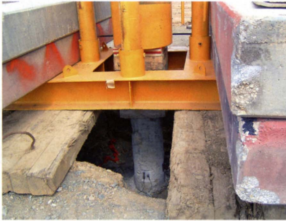
Dynamic load testing at the Brian Lara stadium, Trinidad
