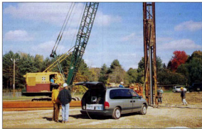
PDA testing on a steel pile.
