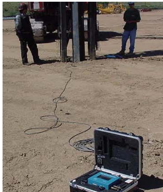
Figure 2. Remote PDA on test pile
