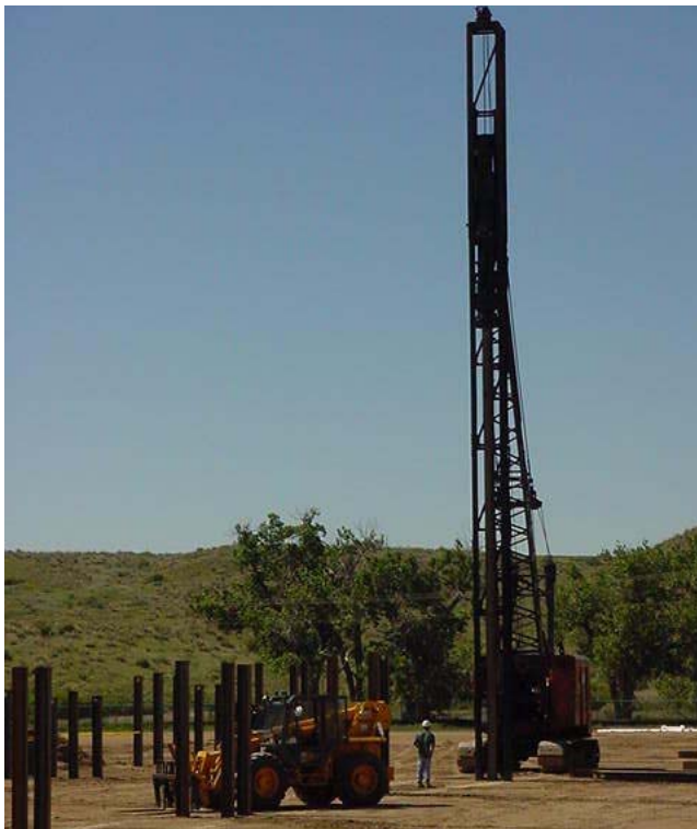
Figure 5. Production piling in progress
