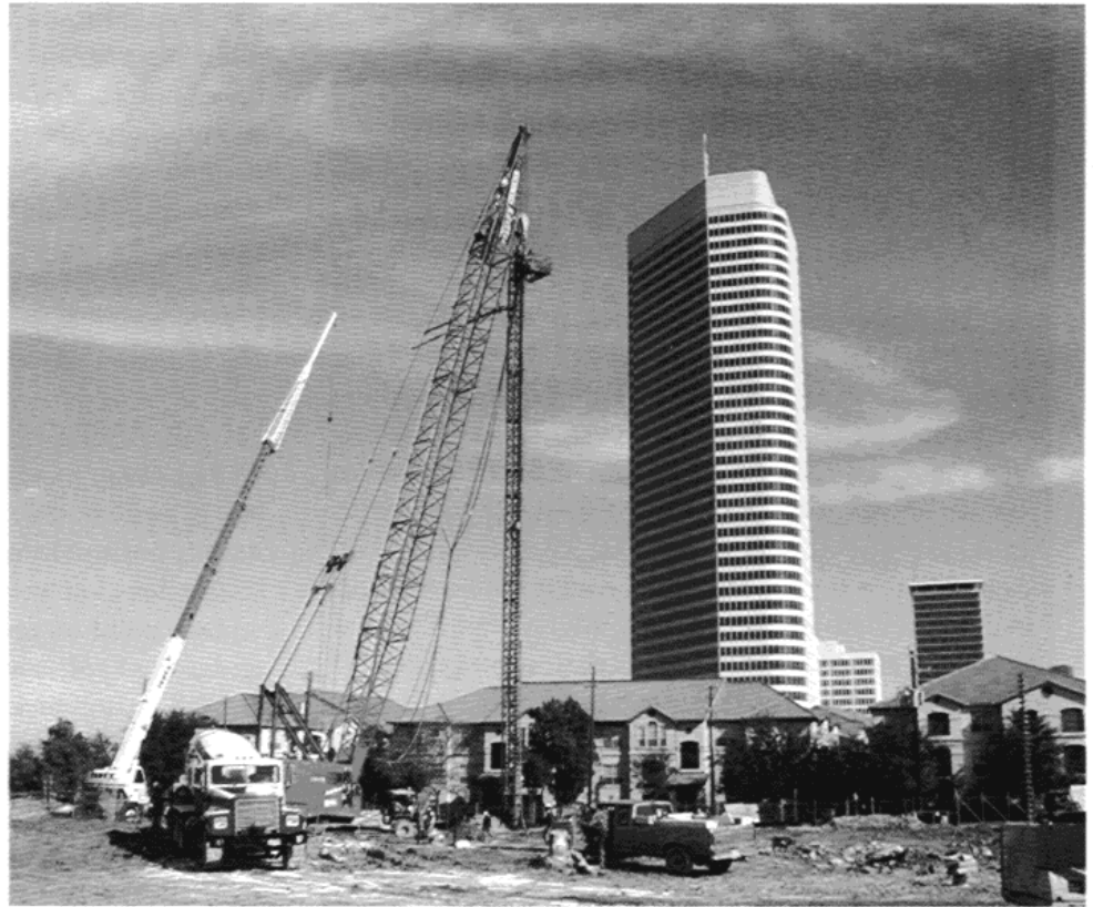
Pile Jobsite, Houston, TX.
