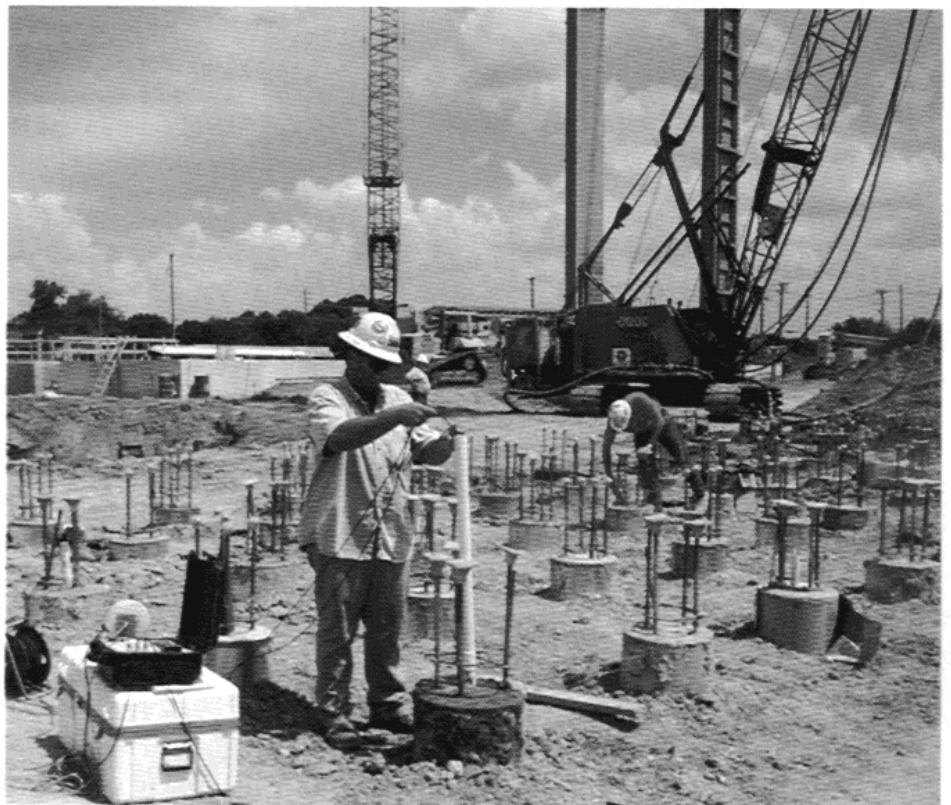
Sonic Integrity Logging.
