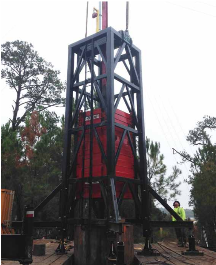
APPLE VIII Load Test System with 60 ton (54.4 MT) drop weight
