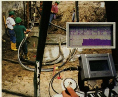
PICTURE THIS Device monitors and records pile installation.
