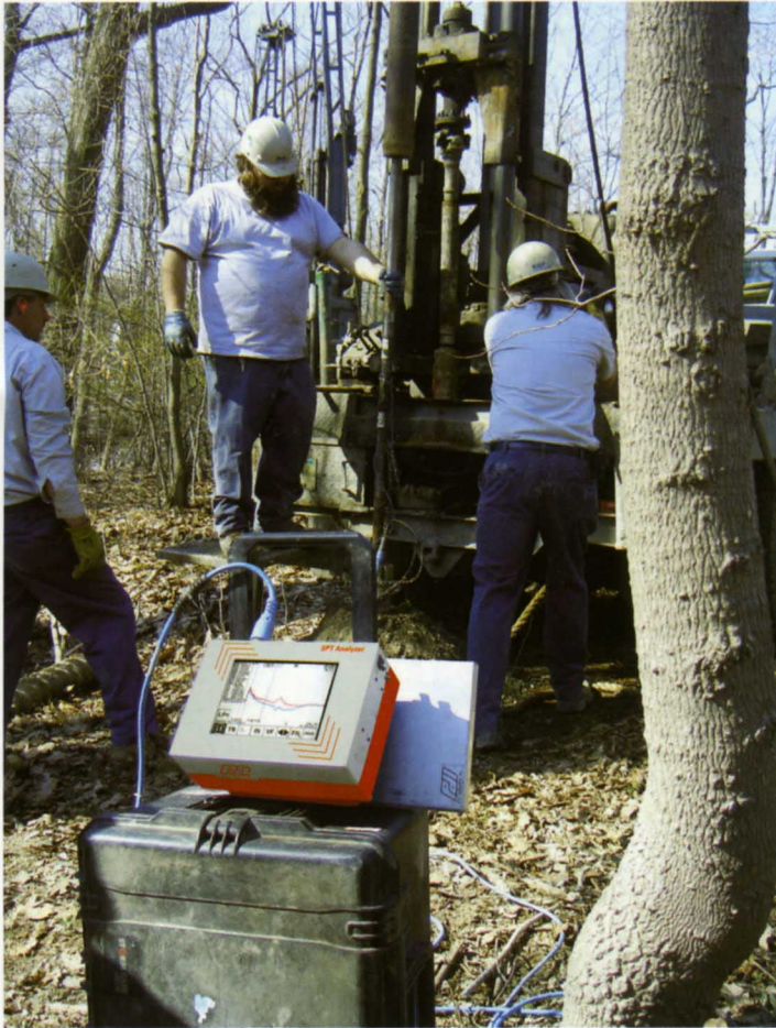
New SPT Analyzer on job site
