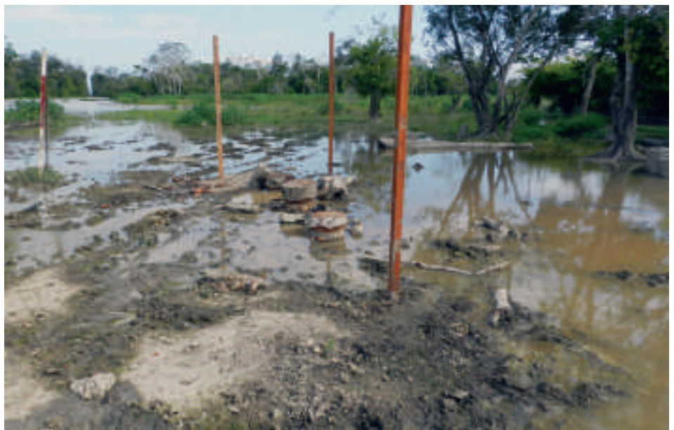
Figure 2. Heavy mud in the dry season makes equipment movement almost impossible
