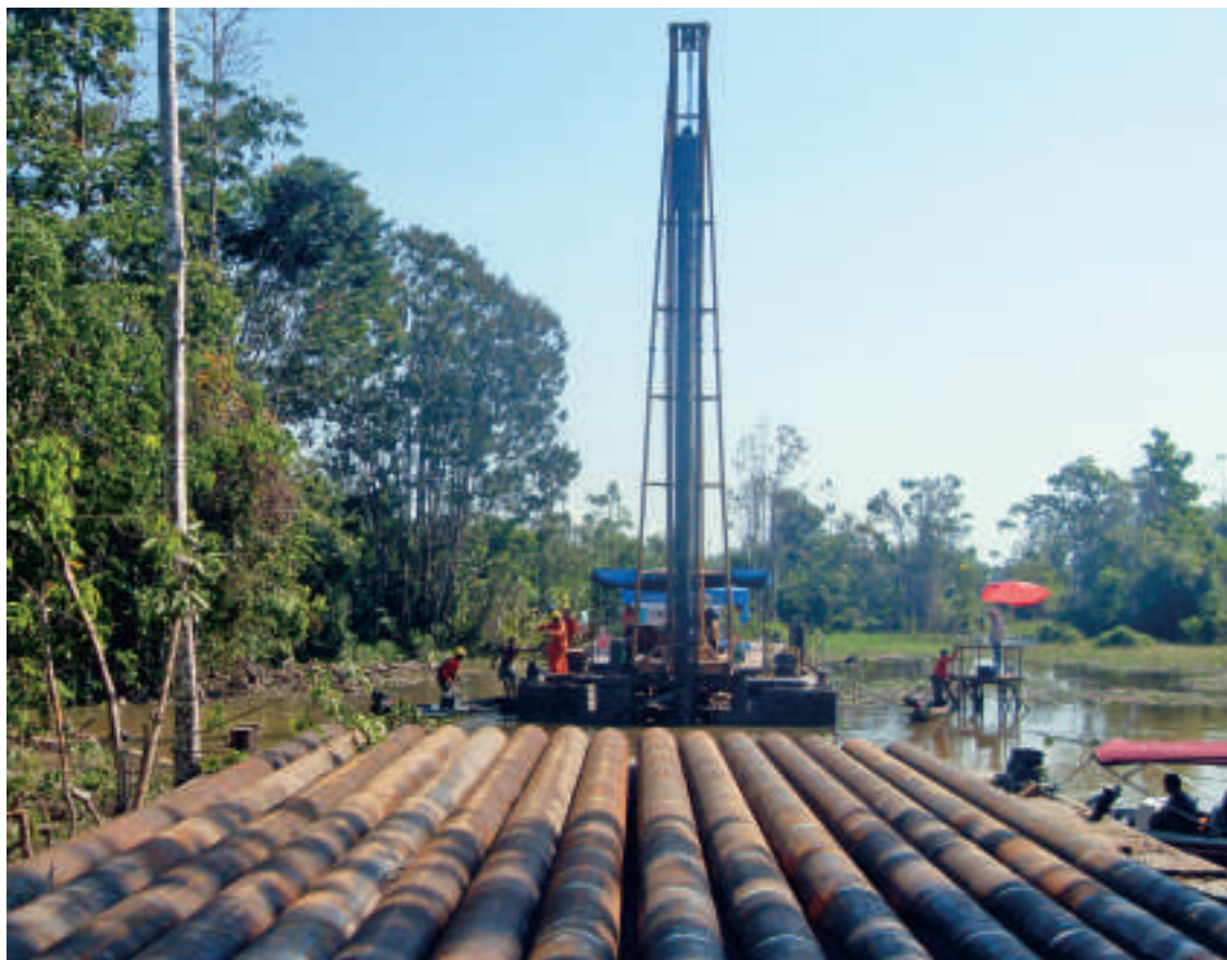
Figure 4. Light gravity driving system, on a small barge
