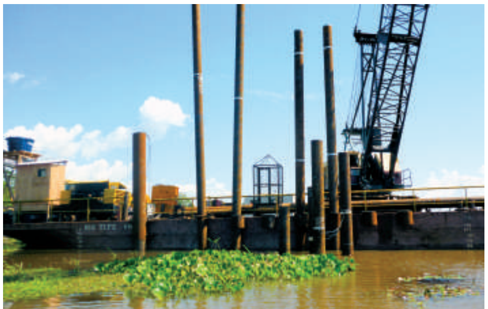
Figure 3. Equipment used for driving the foundations of Tower 238, the “Chinese Tower”
