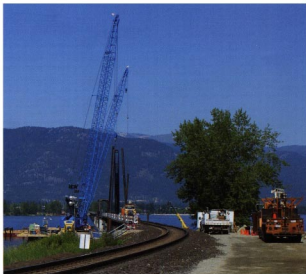
Figure 2: Pile driving on the West End
