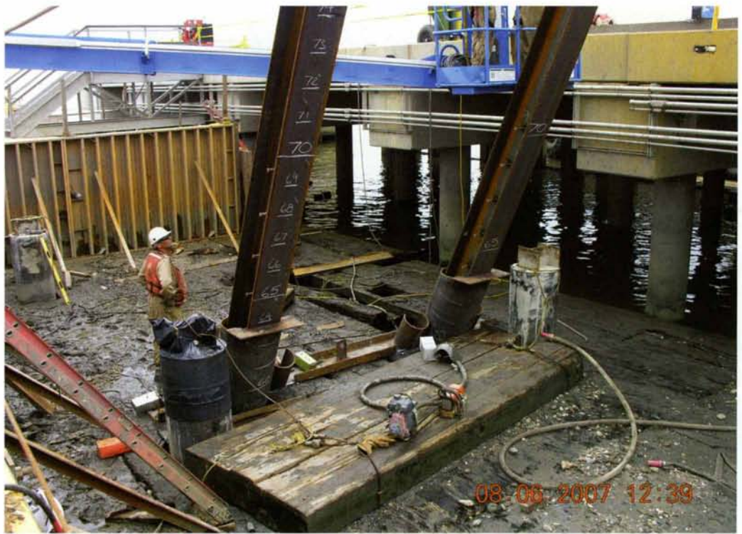
Dock Section B
