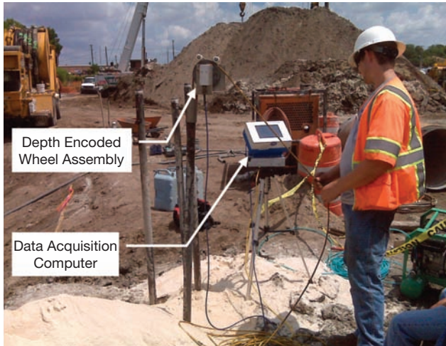
[FIG. 3] Thermal integrity profiler used to assess shaft concrete quality.
