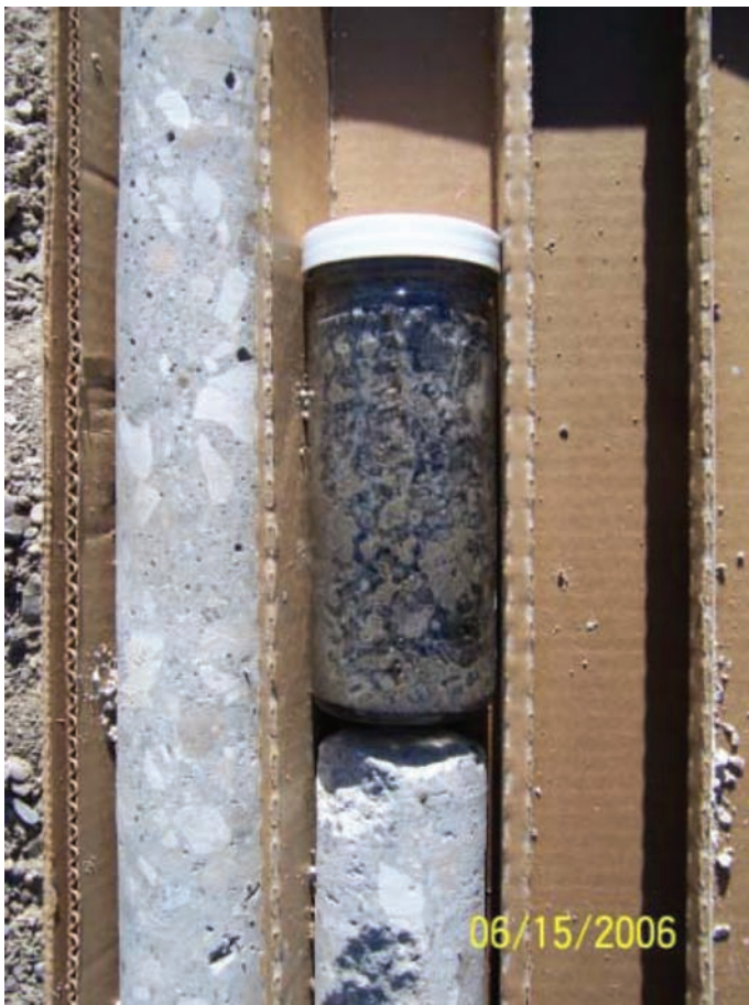
Figure 5. Core from above shaft – sand (in jar) was encountered at approximately 11 m depth.
