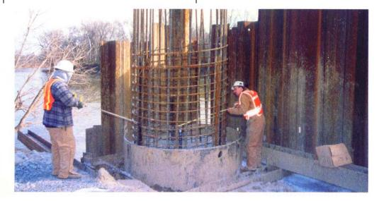
Men from GRL Engineers of Chicago, III check for concrete voids through the use of their Cross Hole Analyzer.
