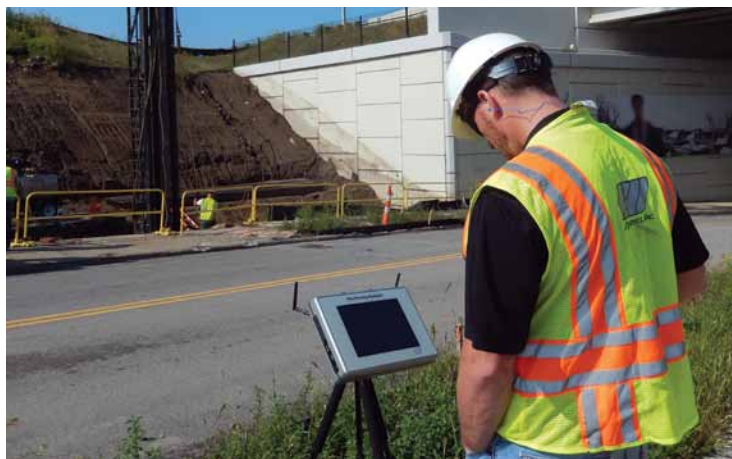
PDA-8G in cantiere
