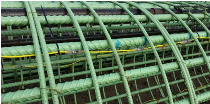
Thermal Wire® cable attached to rebar cage
