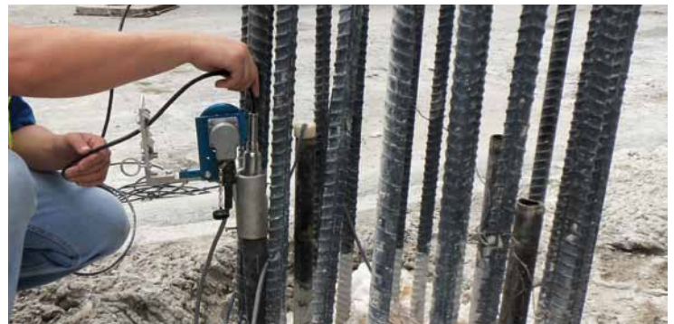
Thermal Integrity Profiler (Probe System)
