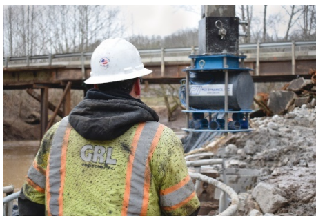
Drilled shaft profile / verticality evaluation being performed by GRL engineer
