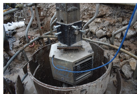
Drilled shaft base cleanliness evaluation being performed by GRL engineer
