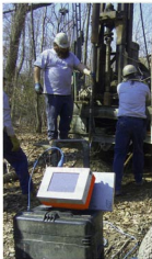
The SPT Analyzer being used on a job site.
