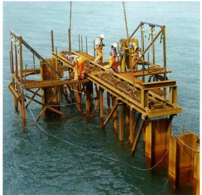
The NZ $22M (€11.6M) design and build contract to extend the wharf involved the design of the piled box, tied and filled with sand to form a mass gravity structure.
