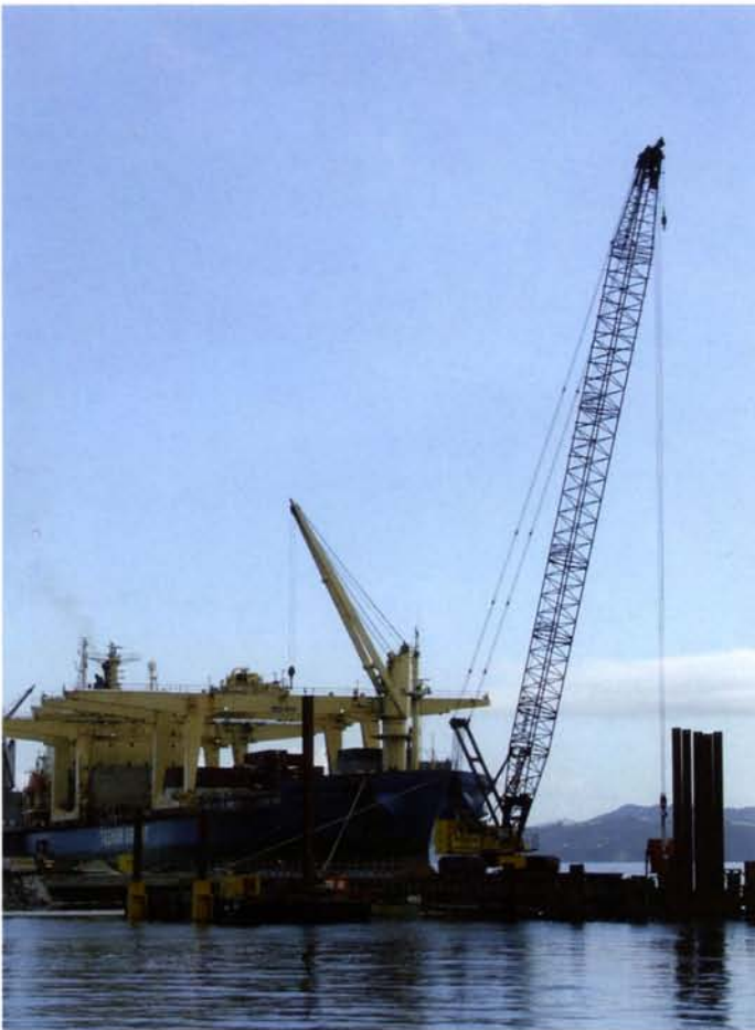
The NZ $22M (€11.6M) design and build contract to extend the wharf involved the design of the piled box, tied and filled with sand to form a mass gravity structure.
