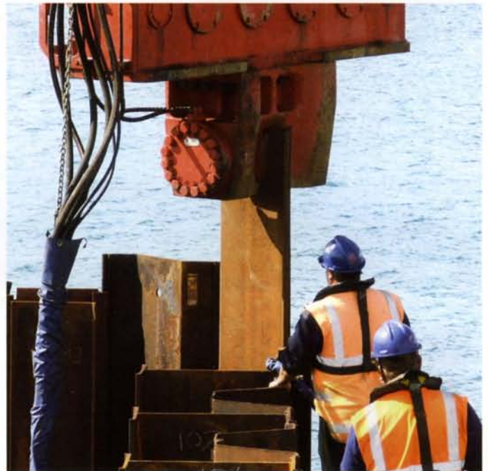
The NZ $22M (€11.6M) design and build contract to extend the wharf involved the design of the piled box, tied and filled with sand to form a mass gravity structure.
