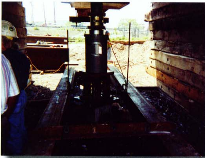
Figure 2: Typical Static (compression) Load Test, New Haven, CT
