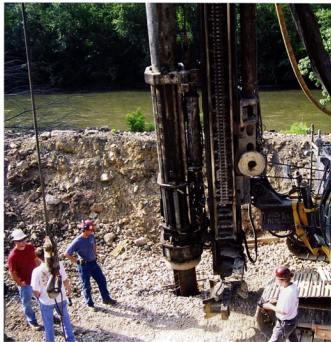
Using the PAK Model Pile Driving Analyzer engineers can gather data from strain transducers and accelerometers attached to piles during the driving process.
