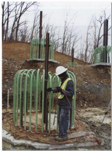
Figure 1 – CSL: Inserting probe into inspection tube.
