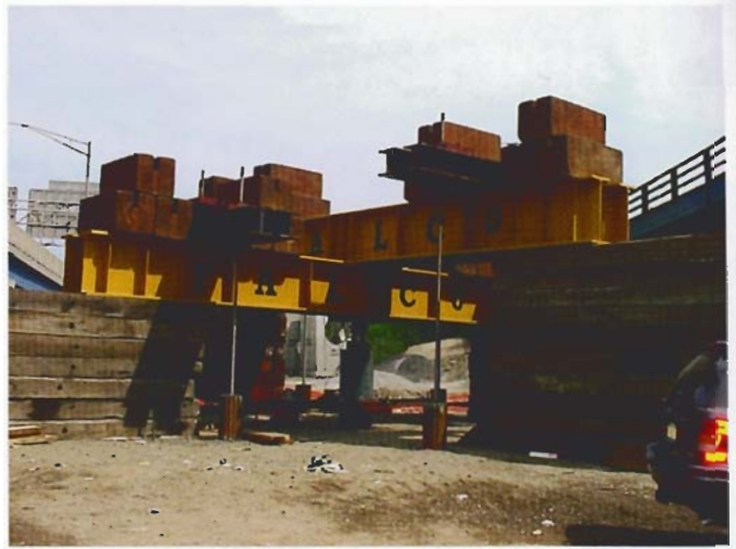
Static Pile Load Test
