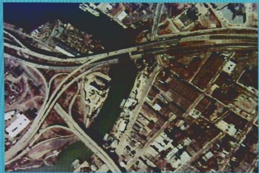
Aerial Photo of Project
