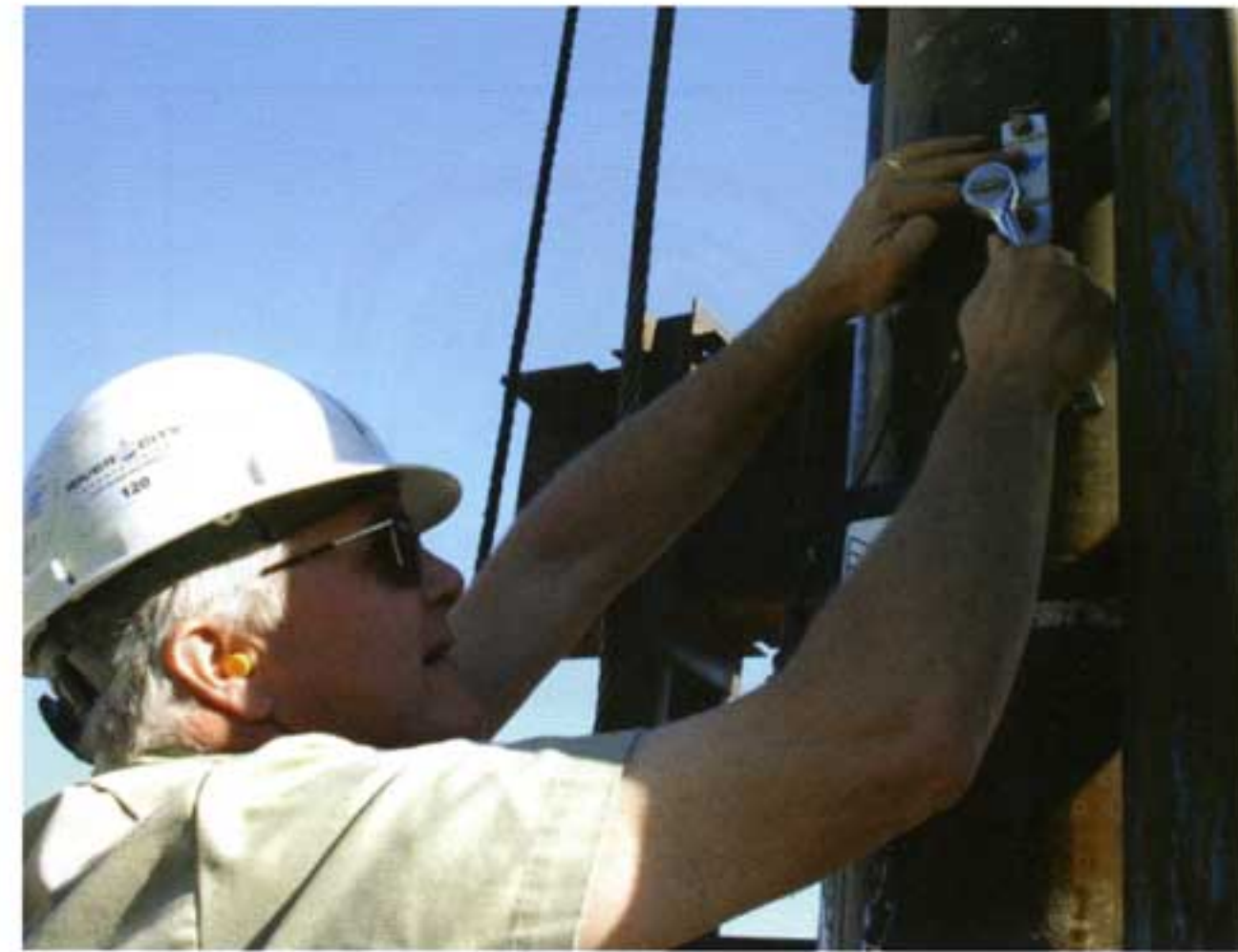
PDPI instructor Pat Hannigan installs wireless gages
