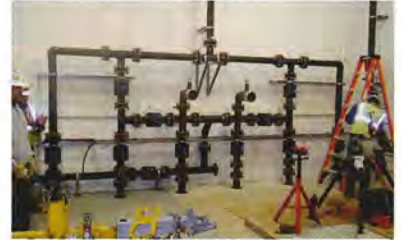
Matt's Underground, LLC installs HDPE piping systems supplied by ISCO Industries.
