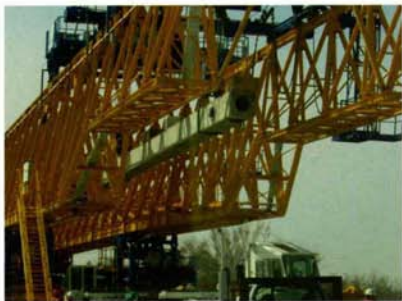
The gantry with the pile at its back end
