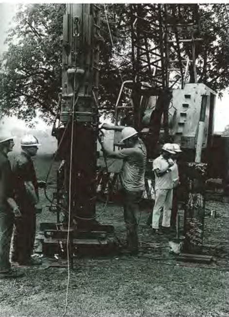
Demonstration of dynamic pile testing, Purdue University, 1972
