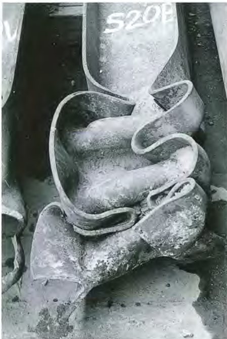
H-piles extracted after overdriving, Sandusky, Ohio, 1975
