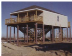
Pearson Piling fiber-reinforced polymer piles are used in coastal areas to elevate house foundations to protect the structures from flooding.
