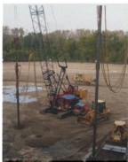
Geotechnology personnel monitor vibrocompaction ground improvement at a Missouri River floodplain site.
