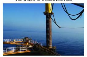
**O**ffshore oil platforms are typically supported by very deep steel pipe piles. These piles must be carefully installed, and should be tested to verify that they can support the load for which they were designed.
