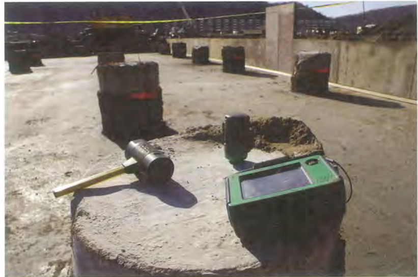
PIT evaluates the magnitude and location of major defects
