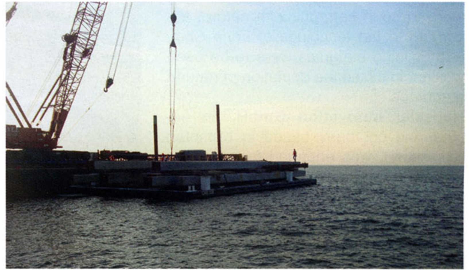
Photos courtesy of Lane Construction Corp.
