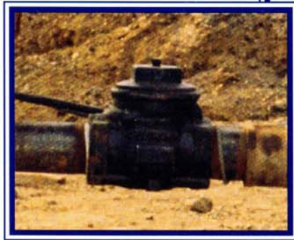
Figure 2. Series 8000 magnetic flowmeter, with a Model IMT25 magnetic flow transmitter
