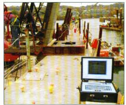
PDA on Charleroi Locks and Dam project
