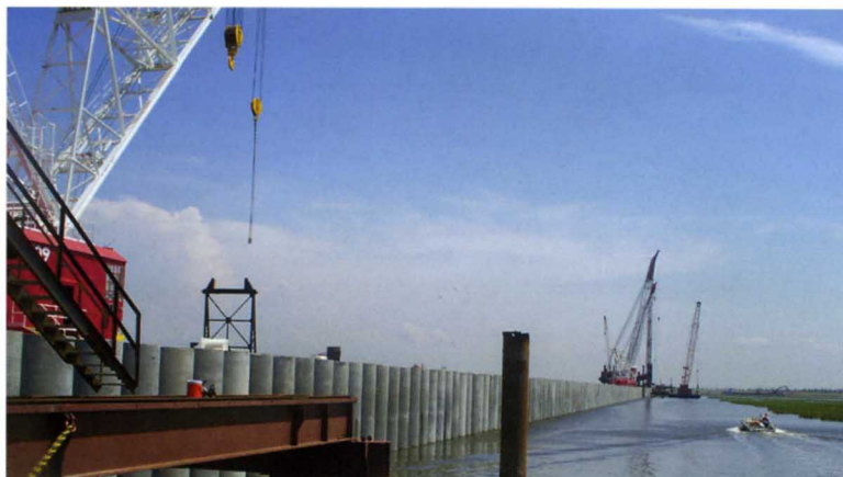
Concrete Cylinder Piles form the New Orleans IHNC Floodwall; Work Trestle in foreground.
