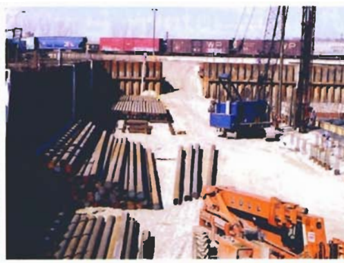
Pile were delivered from the mill by rail in lengths that had been determined by the pre-production pile-testing program.
