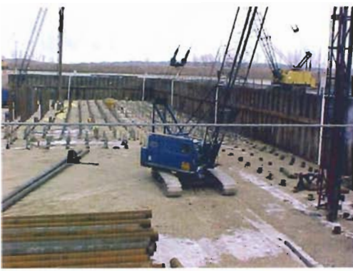
Pile were delivered from the mill by rail in lengths that had been determined by the pre-production pile-testing program.
