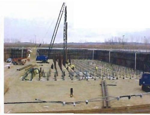
Pile were delivered from the mill by rail in lengths that had been determined by the pre-production pile-testing program.
