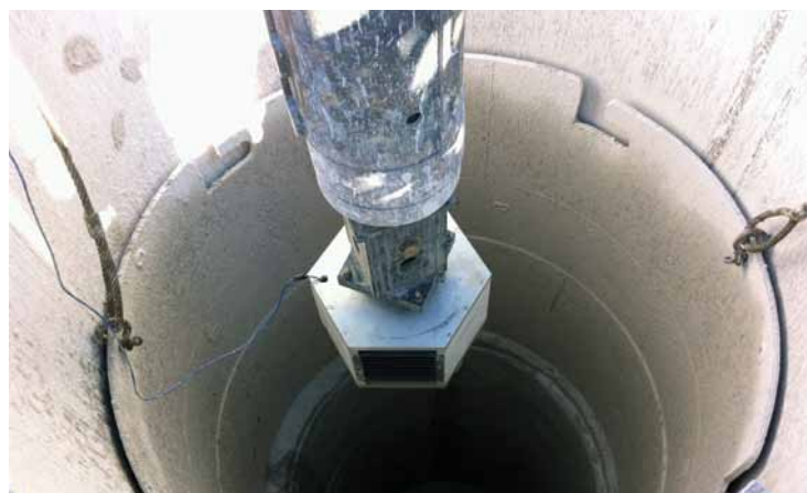
Insertion of SQUID by drill rig into the bore hole
